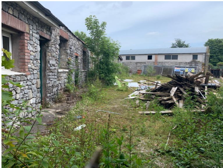
Fig 6. Recolonising vegetation with the courtyard of farm buildings, Phase 2.
