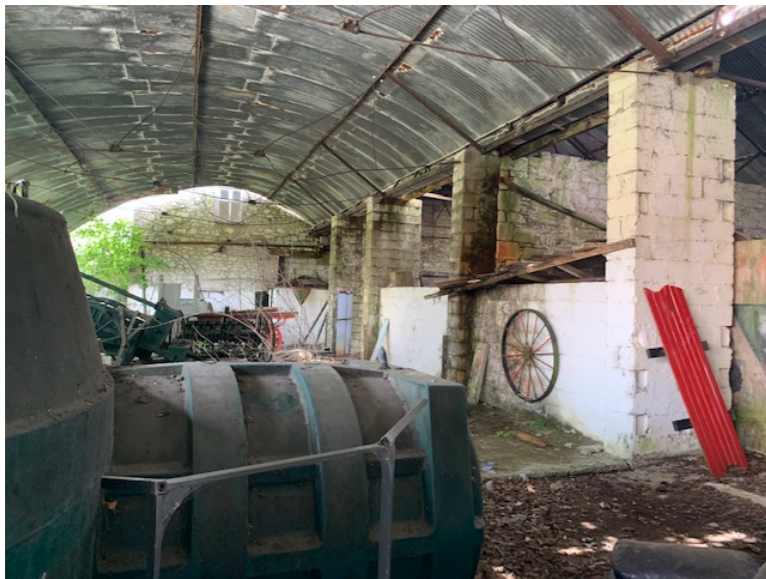
Fig 7. Interior of large barn, Phase 2.
