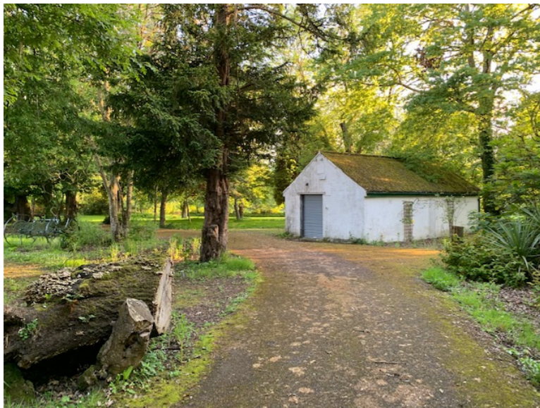
Fig 2. Structures among scattered trees within the walled garden, Phase 2.
